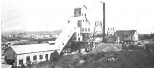
C. SHAFT HOUSE AT NORTH KEARSARGE MINE.
